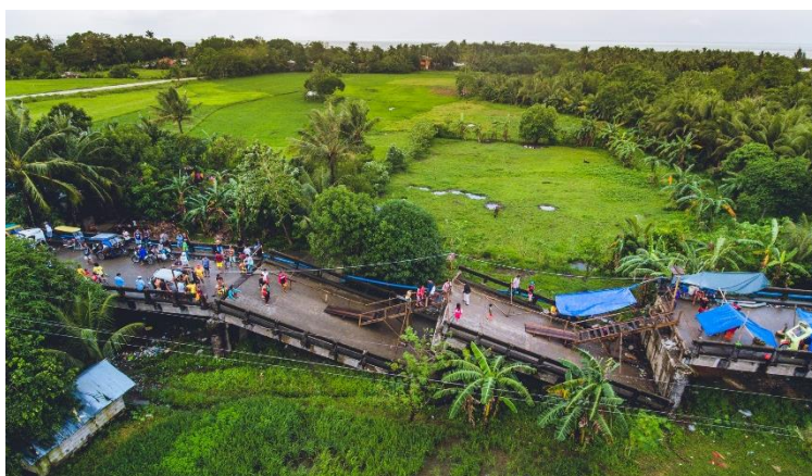
A large part of the Anao-aon bridge, which connects the municipalities of San Francisco and Malimono to Surigao City, collapsed following the earthquake. The state's engineering and construction arm created a series of wooden staircases to create a temporary thoroughfare for the residents.
