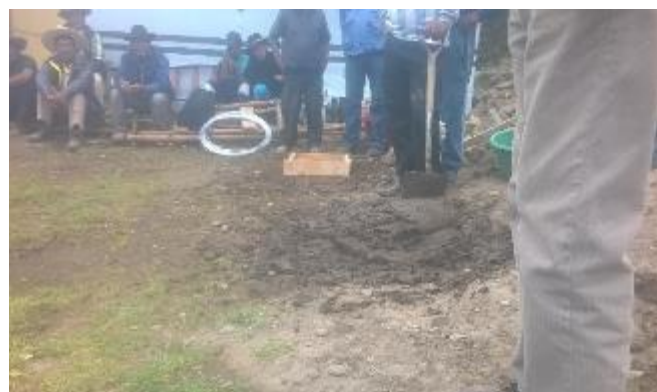
Making improved, earthquake-resistant adobe with the population. Source: PRC
