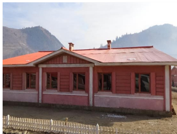
DPRK RCS/IFRC provided CGI Sheets used for construction of new houses at Yonsa County (Photo: Yonsa Branch DPRK RCS)
