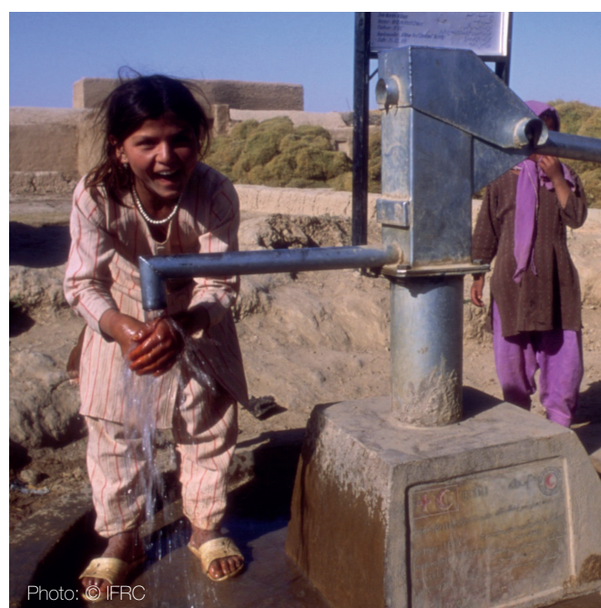
Water pump installed by ARCS.
