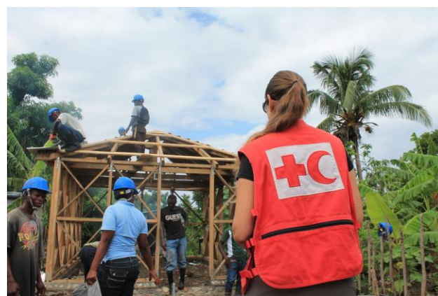
A new shelter under construction in Anse D'Hainault. Source: IFRC
