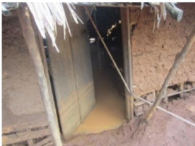
A damaged household in Gemena ©DRC RC
