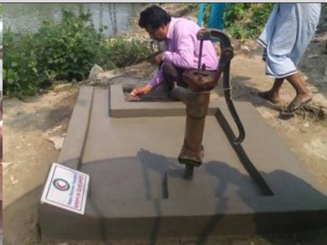
One of the repaired tube-wells in Lakshampur District (Photo: BDRCS)
