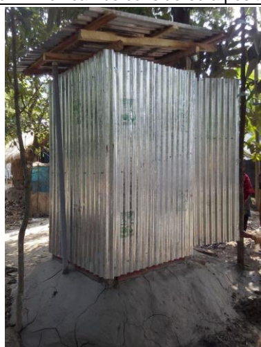
One of completed latrines in Lakshmipur district. (left Photo: Kamrul Hasan, BDRCS) and Leaflet developed by BDRCS and IFRC for owner driven hygiene latrine construction
