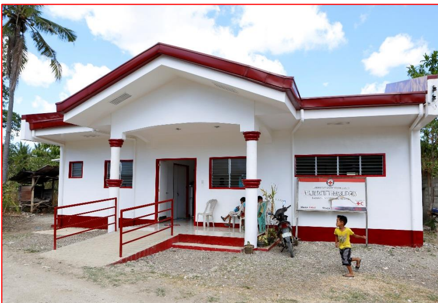
A newly built health facility in San Remigio, province of Cebu, one of the 20 constructed or rehabilitated health facilities by IFRC. The Red Cross partnered with the Philippine Department of Health to reinforce them against future typhoons. Each new facility also received upgrades and additional new equipment. Photo by Cheryl Gaglac/IFRC
