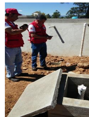
Photo: Quiché delegation, 2017. Carrizal chlorinator tank Source: GRC
