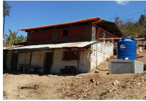
Photo: Community of San Francisco - 2017 Home rainwater collection and storage systems. Source: GRC
