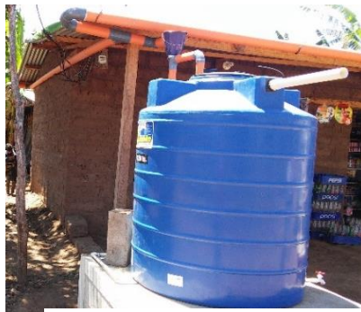
Photo: Community of San Francisco - 2017 Home rainwater collection and storage systems. Source: GRC
