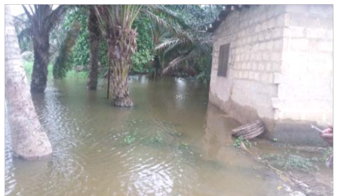
Fig. 2 Flooded house, Weija Community 7Jul
