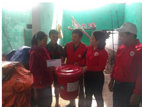
VNRC team visiting an unroofed house in Ky Anh district, Ha Tinh (Photo: Nguyen Vinh Hoa)
