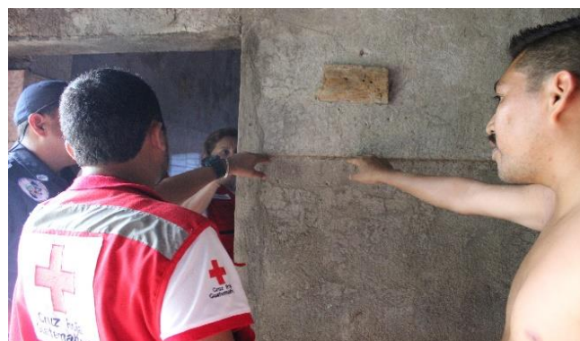
Home flood assessments. Community of Piedad 2. CONRED. Source: DECO/GRC.
