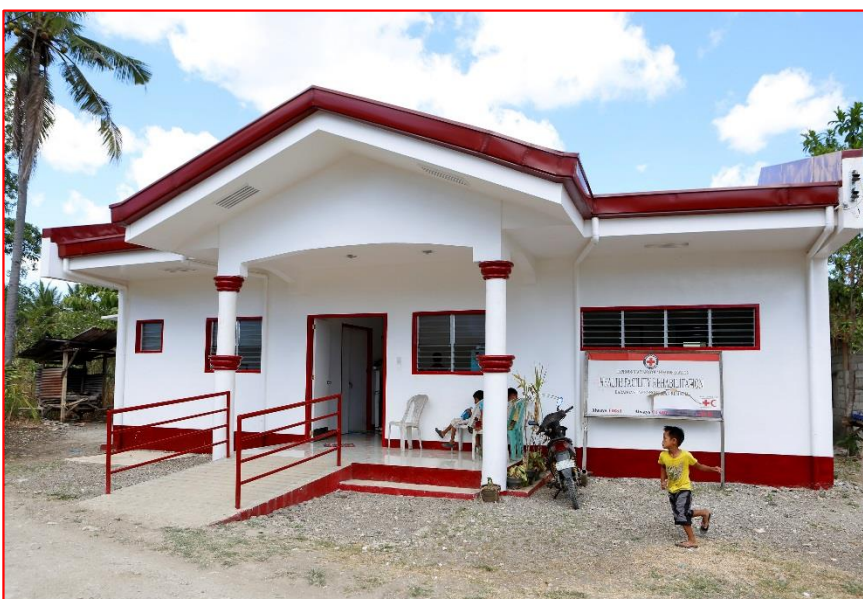
A newly built health facility in San Remigio, province of Cebu, one of the 20 constructed or rehabilitated health facilities by IFRC. The Red Cross partnered with the Philippine Department of Health to reinforce them against future typhoons. Each new facility also received upgrades and additional new equipment. Photo by Cheryl Gaglac/IFRC
