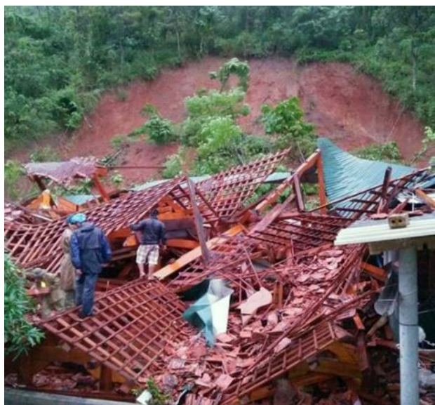
House collapsed in Nghe An province
