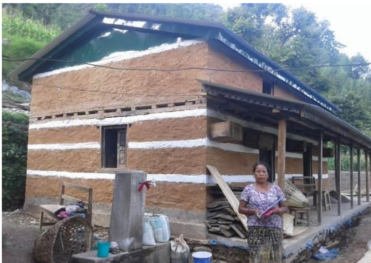
Completed house with the support from NRCS technical assistance and cash grant in Harkapur-2, Okhaldunga District. (Photo: NRCS Okhaldunga District)
