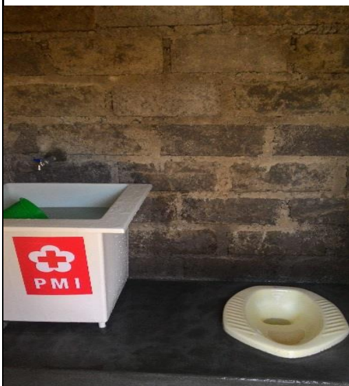
Photo of a rehabilitated latrine with water source for handwashing in Dusun Pegrisngsingan, Tenganan Village (Photo credit, IFRC CCST Jakarta)
