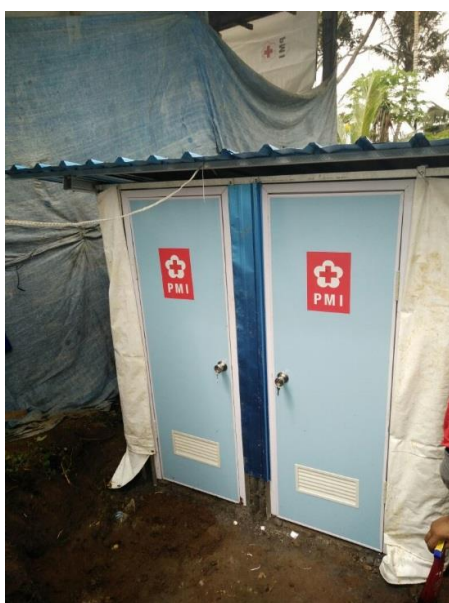
Example of a newly constructed latrine Photo credit: PMI Bali
