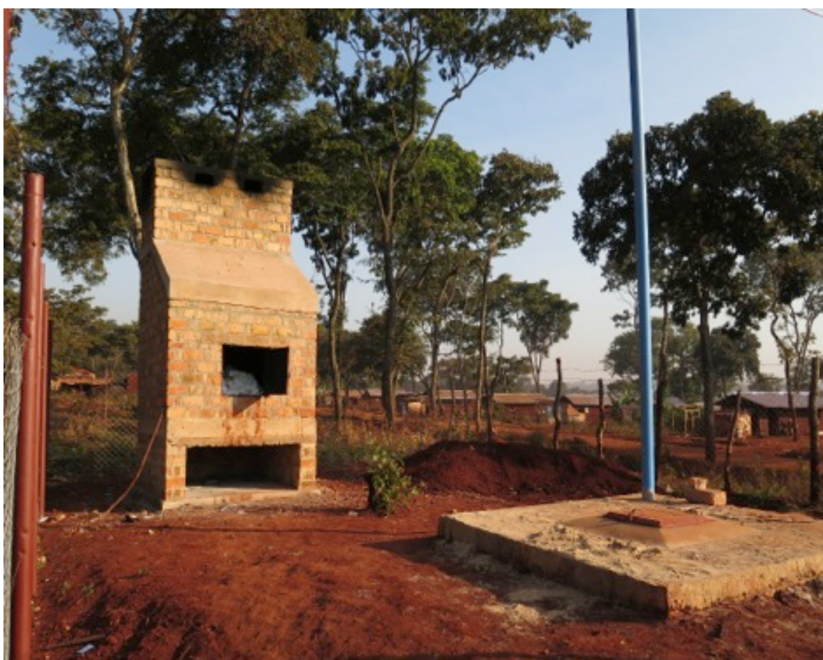
Figure 6: The new Incinerator, Waste Pit, Placenta Pit at Health Post 4, TRCS facility (source IFRC)
