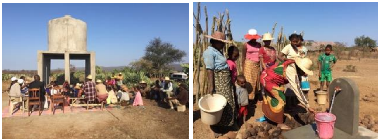
Left: Group discussion in Mahatalaky; in the background, a newly constructed water reservoir with a capacity of 20m 3 . Right: One of the operational water points in Berano Fokontany.
