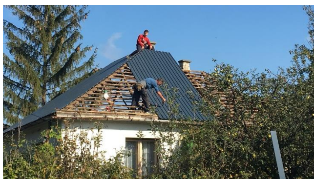
Image 2. Damaged roof being repaired. Photo: HRC
