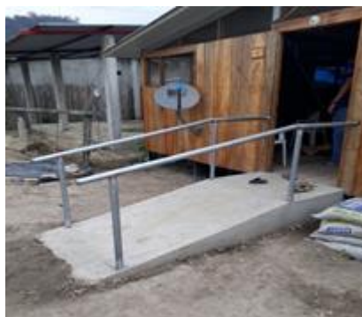
Access ramps improve habitability conditions in the progressive shelters. Source: ERC.
