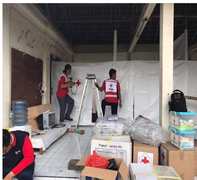
PMI volunteers used tarpaulins as walls and partitions turning community spaces (Banjars) into evacuation Photo credit: PMI Province Bali
