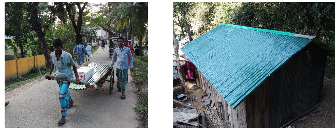
Beneficiaries returning home with their CGI sheets after receiving them from the Bandarban BDRCS district branch ( Left Photo: IFRC ). One of the beneficiaries house in Naikhongchari sub-district of Bandarban has its roof repaired using the given CGI sheets ( Right Photo: IFRC )
