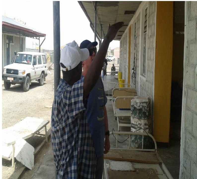
Renovation of Bidu Health centre. Source: IFRC
