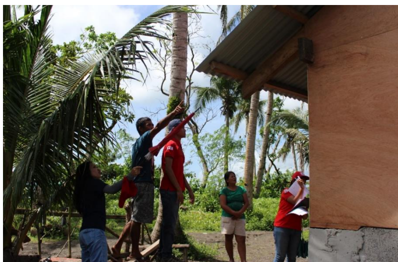
Red Cross volunteers continuously monitored shelter repairs to ensure that the safe shelter principles were observed. Volunteers also acted as a channel for communication between the chapter and the beneficiaries, taking note of feedbacks from the community and delivering responses of the chapter, (Photo: PRC/IFRC)
