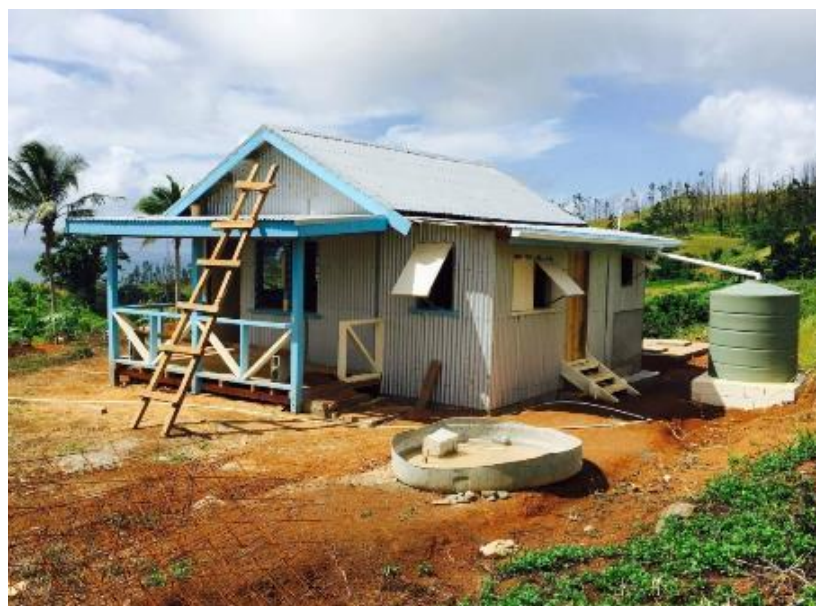
Demonstration Shelter Model in Delaikuku in Tailevu. April 2017. (Photo: FRCS)
