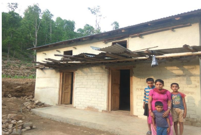
After: Toyanath Parajuli's family in front of their newly constructed earthquake resistant house. (Photo source: NRCS Okhaldhunga District Chapter)
