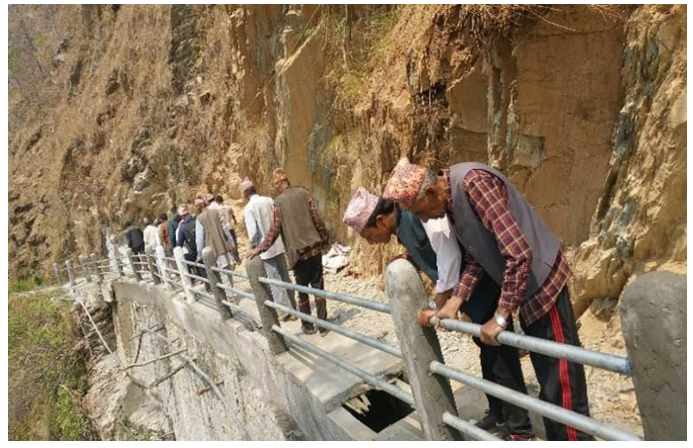
After construction of brest wall. (Photo source: NRCS)
