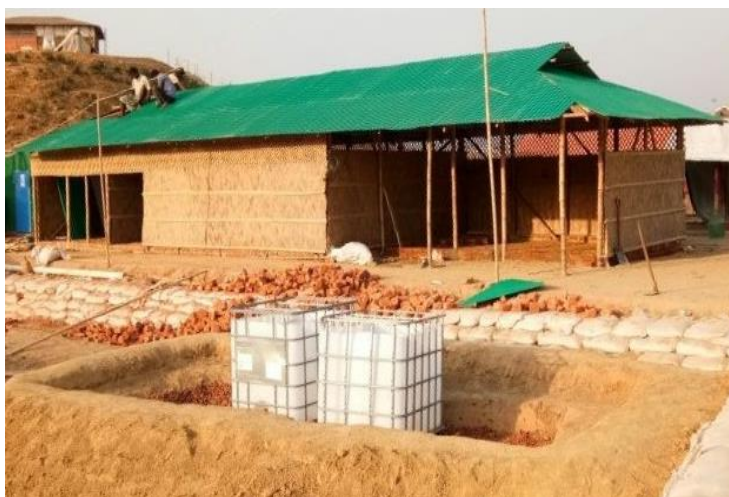
Faecal sludge infrastructure under construction (Photo: IFRC)
