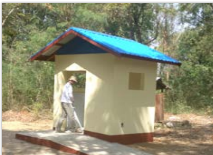
Figure 5 - A school toilet in Budalin Township, adapted for disabled access
