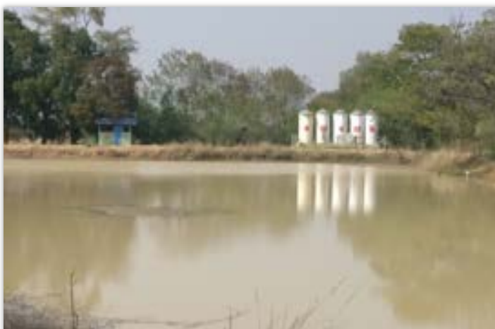
Figure 4 - Red Cross water system behind community water source pond in Wundwin Township, Myanmar
