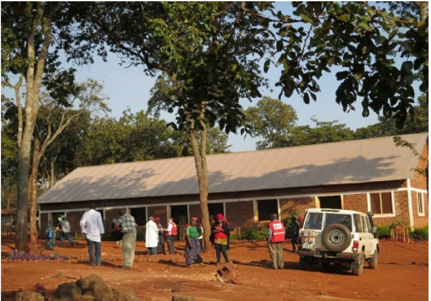
The Red Cross health care facility in Nyarugusu (source IFRC)
