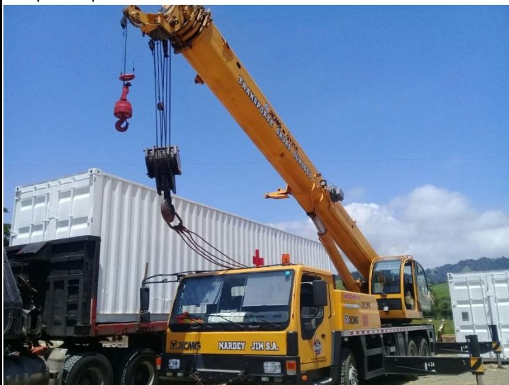
Appeal funds were used to refurbish the containers that had contained housing materials from the Spanish Red Cross in warehouses with pre-positioned NFIs. Source: ERC.
