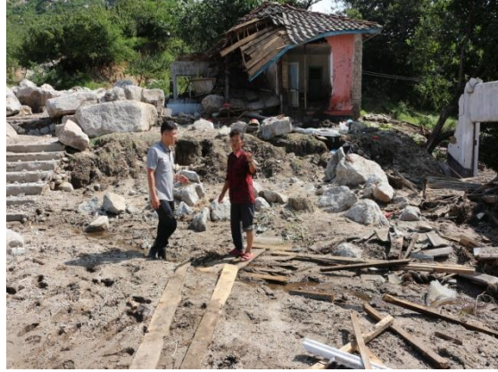
NDRT member is conducting needs and damage assessment. (Photo: DPRK RCS)
