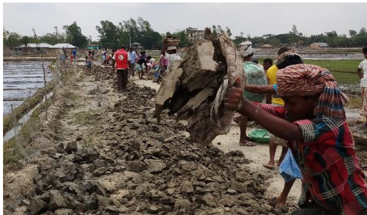
Earthen road repairing by beneficiaries at Banskhali, Chattogram district. (Photo: IFRC)
