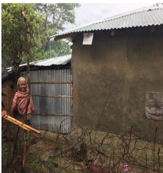
Repaired roof in Banskhali village
