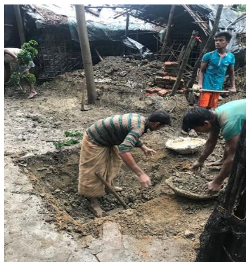
Deep tube well digging in Banshkhali
