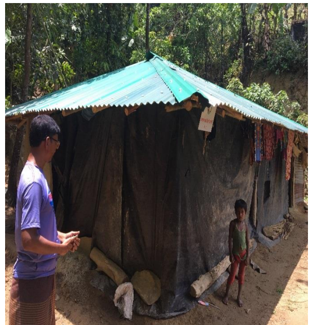
Repaired house in Naikhongchari
