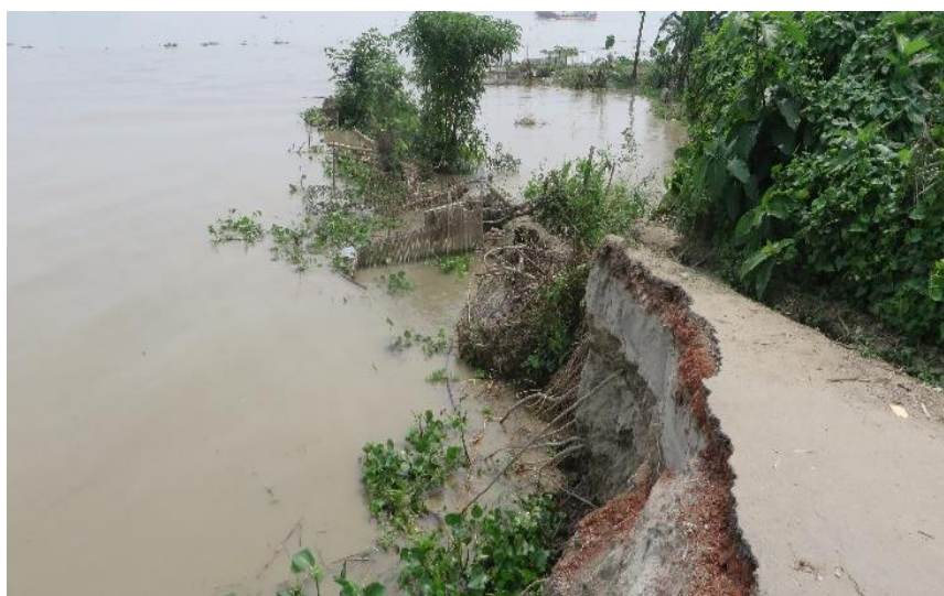
Due embankment collapse caused by riverbank erosion, agricultural land, homestead and even infrastructure like pavement road have been washed away in Shariatpur district. (Photo: BDRCS)
