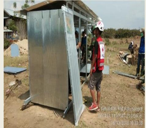
PMI is constructing latrines and bathrooms for the community. (Photo: PMI)
