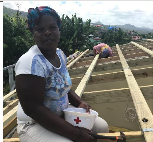
A DRCS volunteer repairs a damaged roof. Source: IFRC
