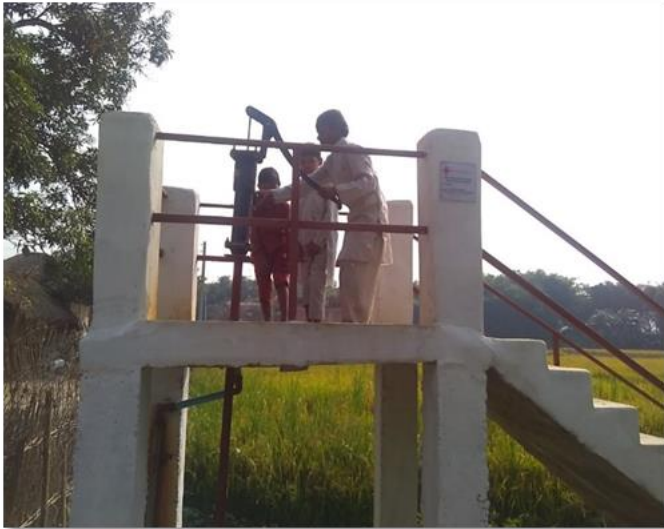
Elevated tube well constructed in Hanumannagar Kankalini-14, Saptari district (Photo: NRCS)
