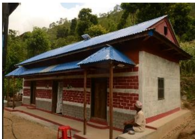
One of the owner driven houses constructed with the Red Cross shelter cash grant support in Sindhuli district. (Photo: NRCS)
