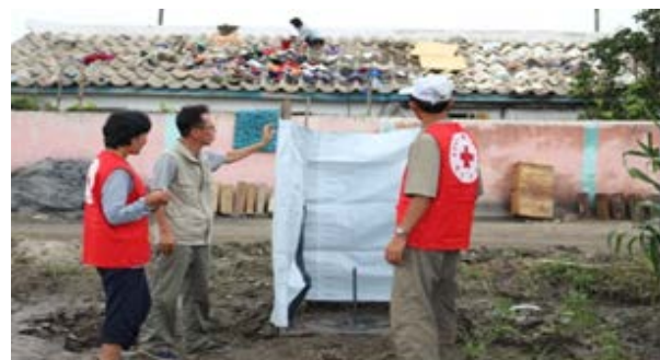
Building temporary latrines, September 2018. (Photo: DPRK RCS)
