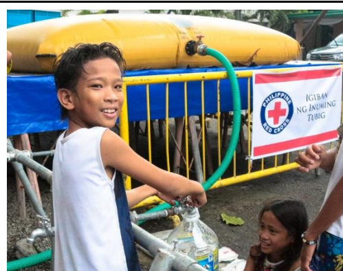
A child fetches a water from the tap stand set-up by PRC to provide the water needs of the affected population. A total of 11,216 people was reached with safe drinking water support. (Photo: PRC)
