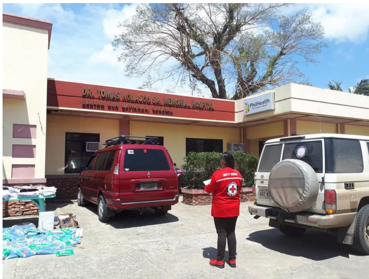
PRC assess the condition of Dr Tomas Nolasco Sr. Memorial Hospital in Cagayan. Based on the RDANA, damages were reported in health facilities but were still functional. (Photo: PRC)
