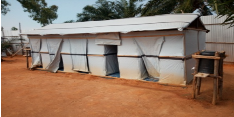
Figure 2 fully constructed latrines at Rumonge refugee site
