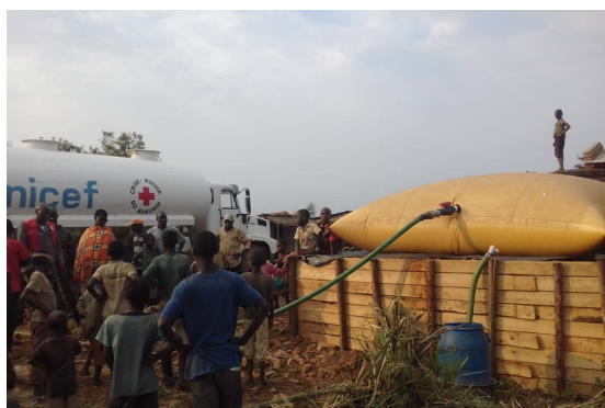
Figure 3: Launching of a bladder tank
