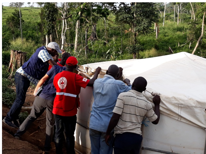
Photo: Verification sedimentation process at Maratatu Water Treatment Unit
