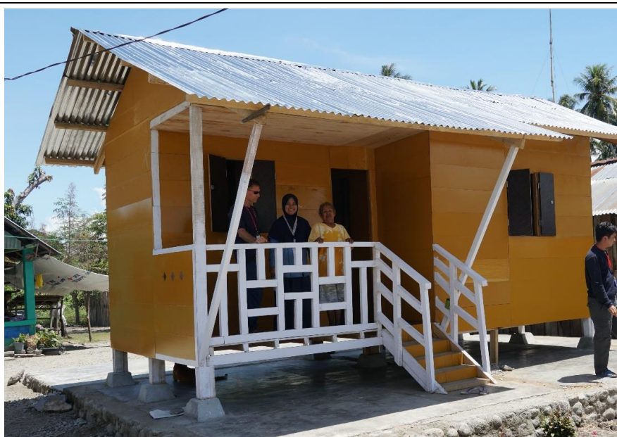
One of the transitional shelters constructed in Sambo village in Sigi district. Construction of 40 transitional shelters was supported by a surge shelter delegate deployed for the operation. (Photo: IFRC)
