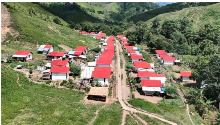
Relocated families begin to start anew in their new shelters. With the support from the local government, beneficiaries were able to secure land where their new shelters are established. (Photo: PRC/IFRC)
