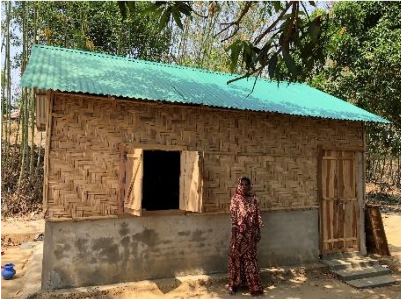
Newly constructed shelter at Telar khola, Gayalmara village (host community). Thanks to the financial contribution from OFID. (Photo: BDRCS)
