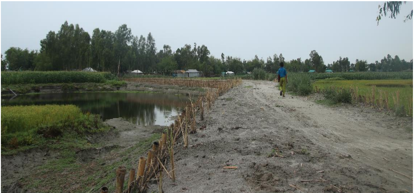
Earthen road repaired in Lalmonirhat under the DRR activity. (Photo: BDRCS)
