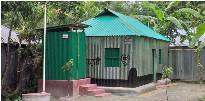
One of the beneficiaries installed a latrine as per DPHE design and rebuilt their house considering PASSA findings after receiving the shelter & latrine grants from BDRCS in Lalmonirhat District. (Photo: IFRC)
