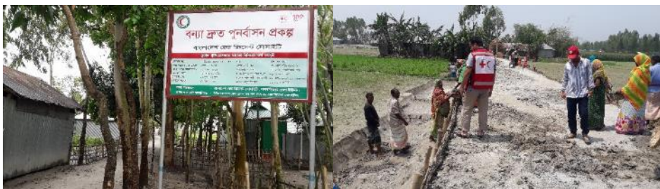
Small scale mitigation work through cash for work (CfW) in the community. (Photos: IFRC)
