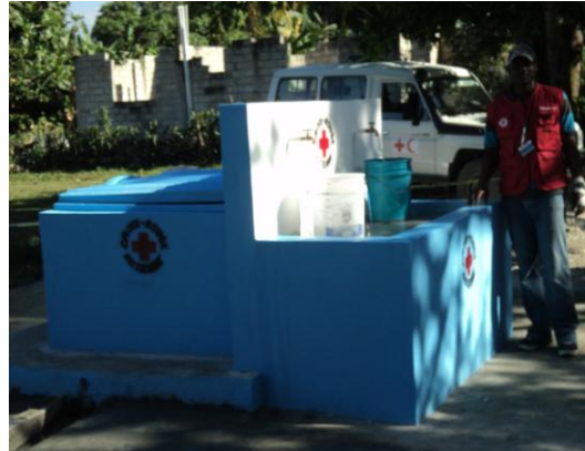
The borehole after rehabilitation/IFRC
