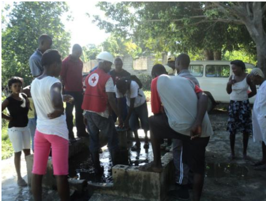
A borehole under rehabilitation in Léogâne. IFRC
