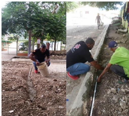
Photo 10: Ditch digging and pipe installation – Guayabal. Source: DRC 2018.
