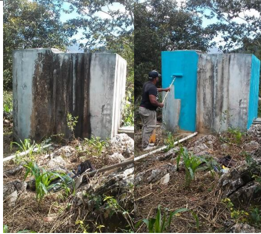
Photo 9: Reconditioning of distribution system – Los Bolos. Source: DRC 2018.
