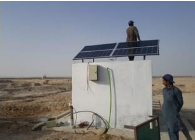
Left – installation of solar water pump by workers. Right – completed solar water pump station. (Photo: PRCS)
